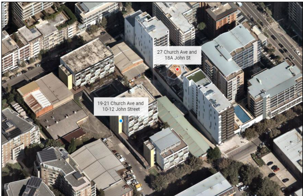
Figure 6 – Aerial view identifying neighbouring sites Source: Statement of Environmental Effects
