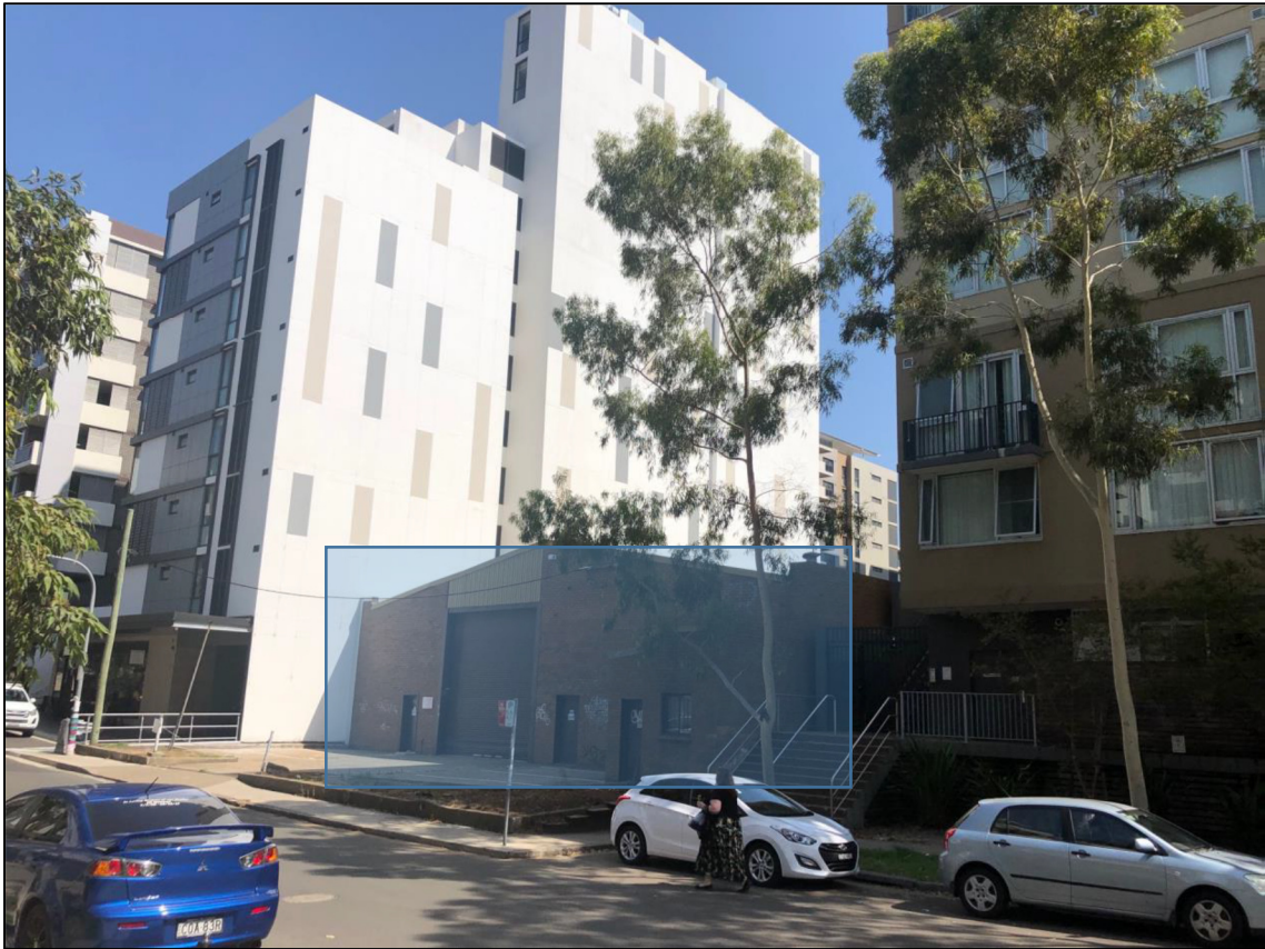
Figure 2 - Existing warehouse at 16-18 John Street
